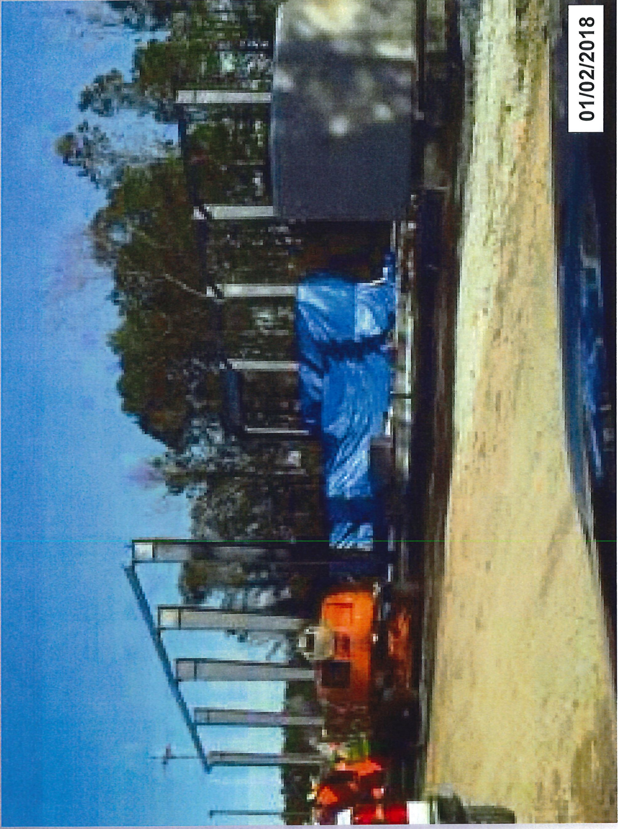
Gensets covered with tarps, erection of building begins, 12,000 gallon fuel tank is placed in right portion of photo
