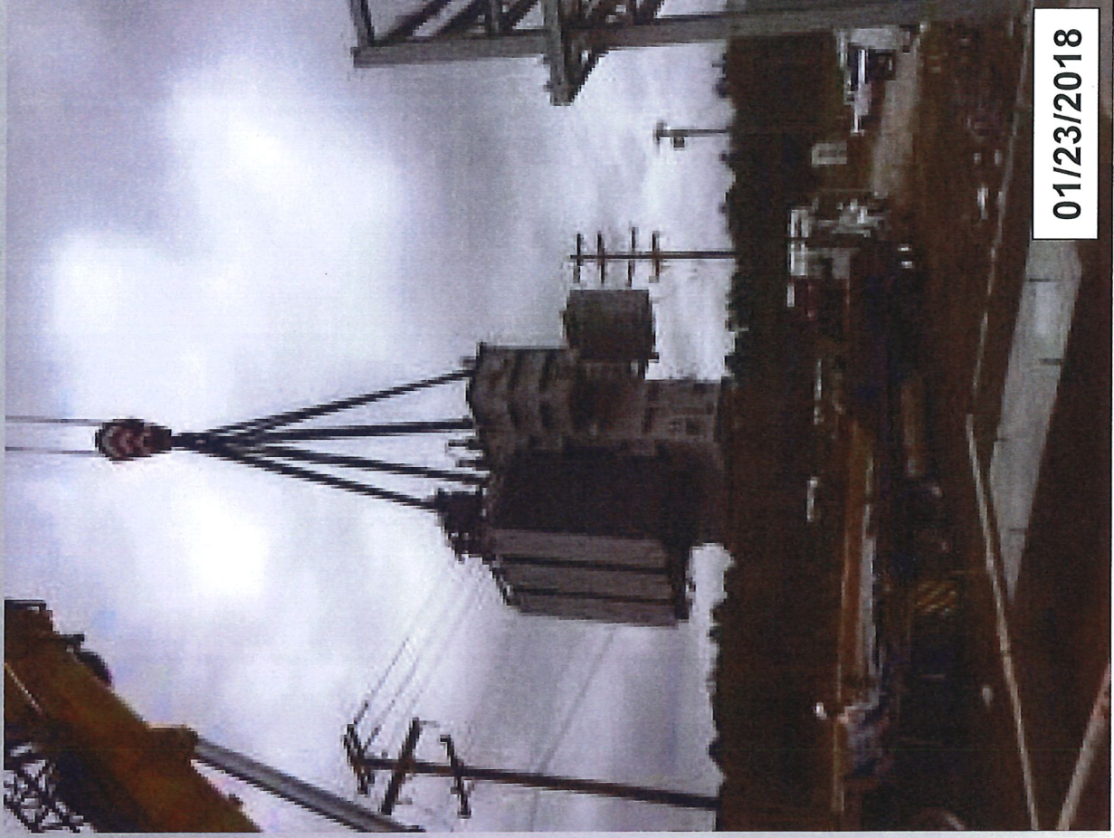
Placement of GSU transformer and spare
