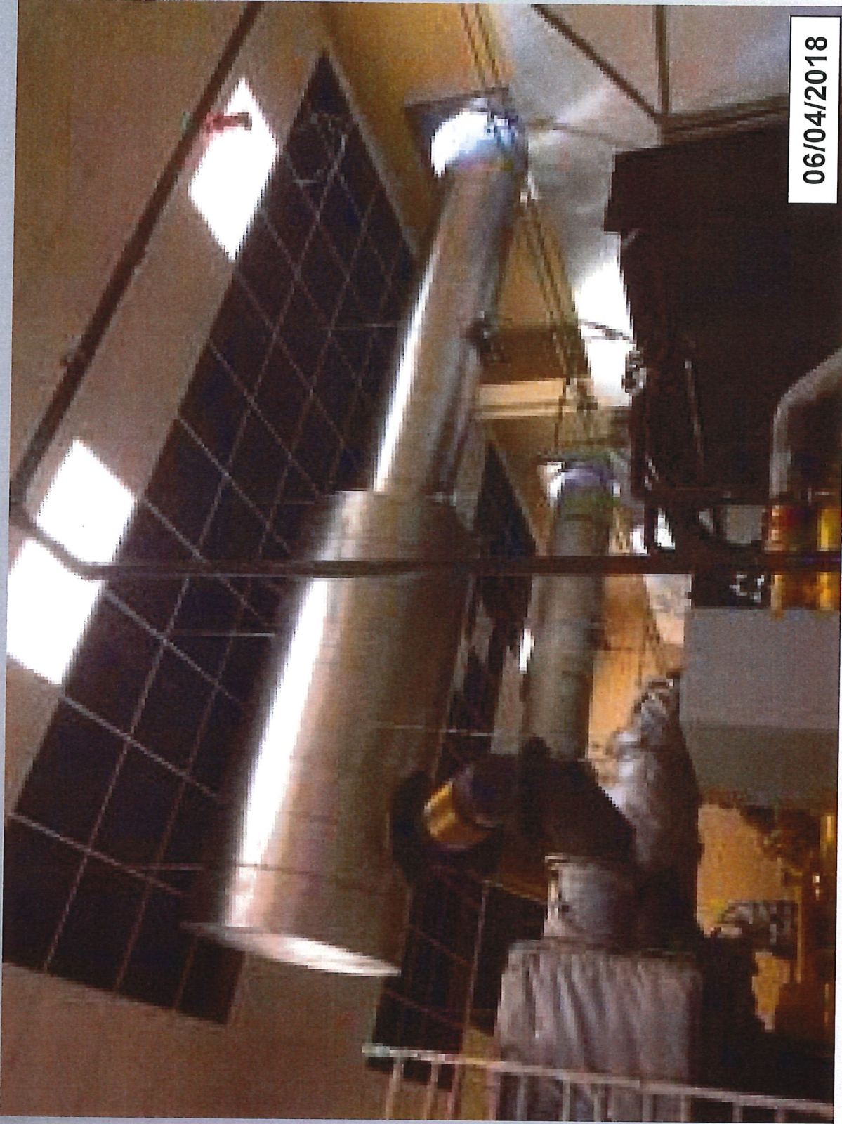
Insulation placed around muffler/exhaust
