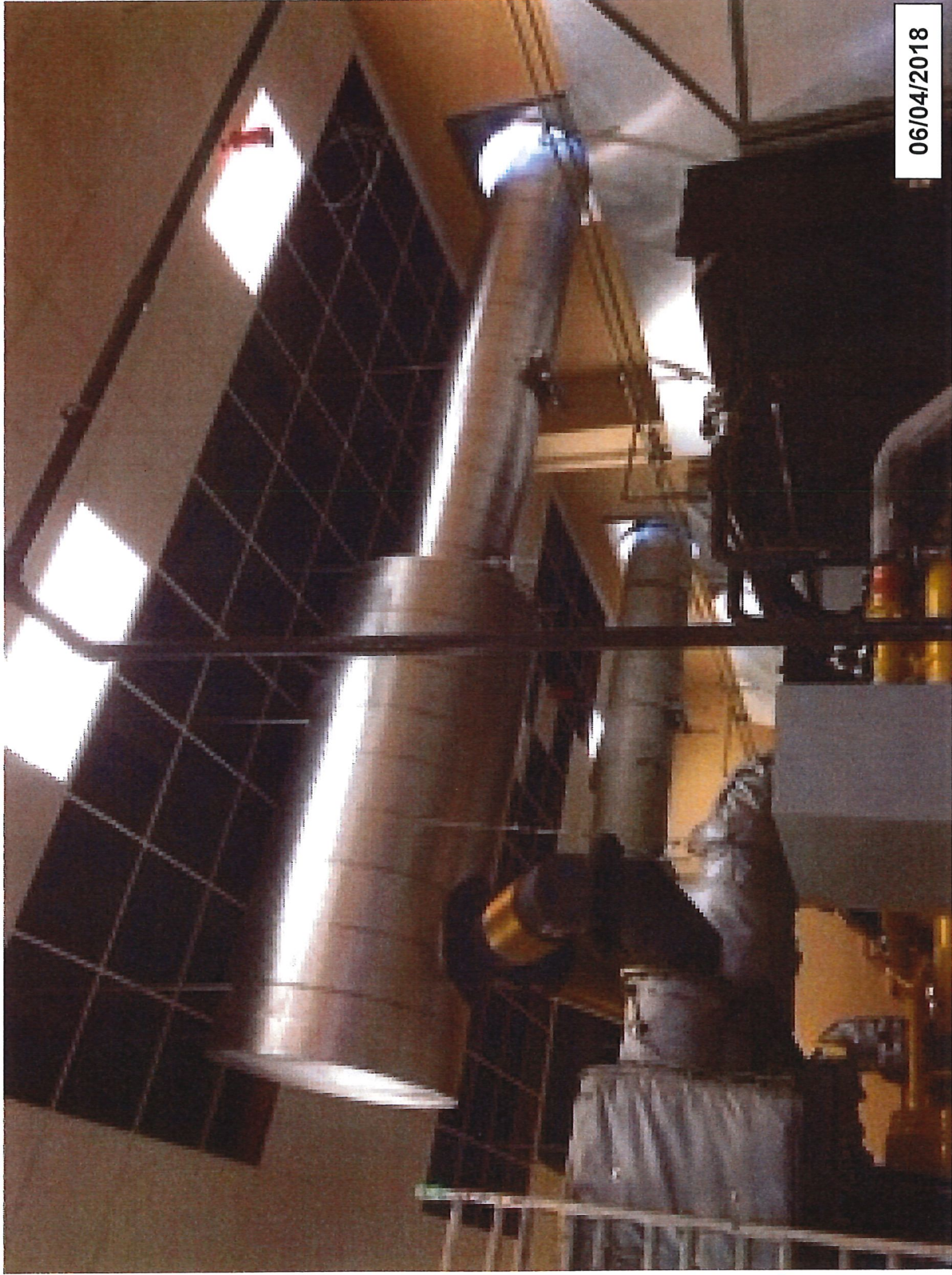
Insulation placed around muffler/exhaust
